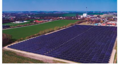
14.5 MW collector field intalled on a former industrial site
