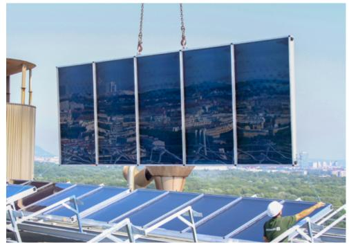
Installation of large flat plate collectors with 13 m<sup>2</sup> each on the roof of the boiler house. Due to the low inlet temperature of 20 °C into the solar field, the collectors achieved a high specific annual yield of 688 kWh / m<sup>2</sup> in the first year of operation.
